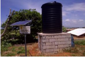
The new solar pumping system provides energy to move water from the concrete storage tank to two elevated plastic tanks
